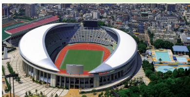
Big Dome Rooftop Control
